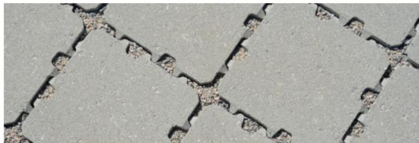
Figur 0.1 – Permeable belegningsstein i betong
